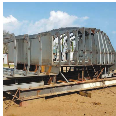
The steel power tug starts to take shape at Marine Inland Fabricators yard in Panama City, Florida.
