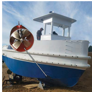
Nearing completion, the 12-inch steel thruster tube can be seen in the hull.
