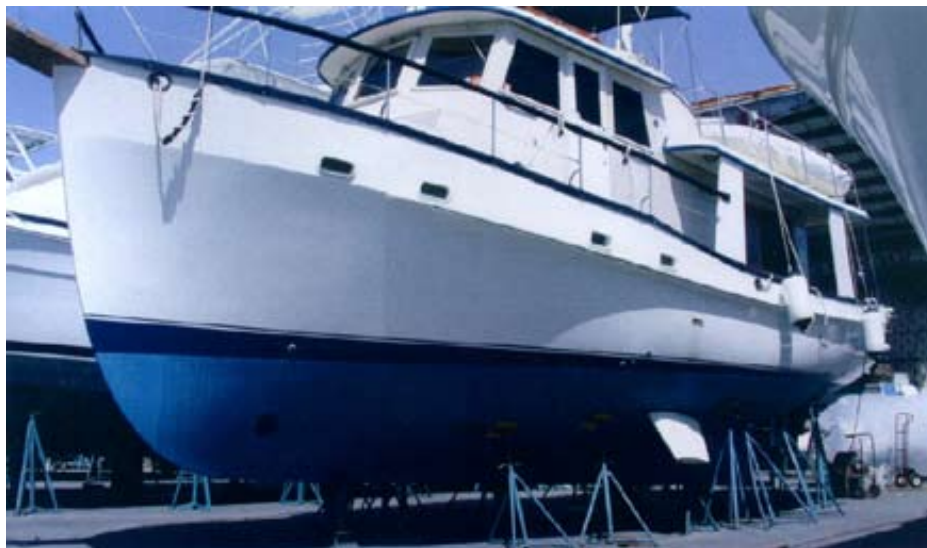
The 42 foot 'Avalon' during installation of WESMAR stabilizers and new Vortex bow thruster. Photo courtesy of YEP, Fort Lauderdale
